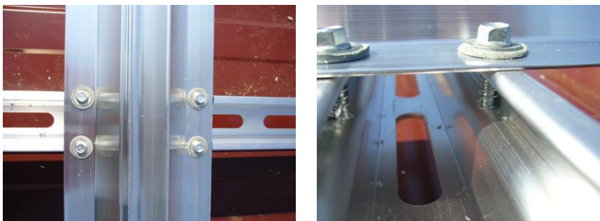
Figure 24 Base profile fastening to C-rails
