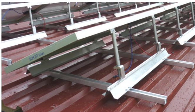
Figure 17 C-rail as lower level of the cross rail assembly
