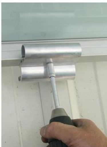
Figure 10 Mounting the back (left) and front (right) module bracket set
