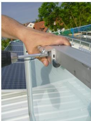
Figure 10 Mounting the back (left) and front (right) module bracket set
