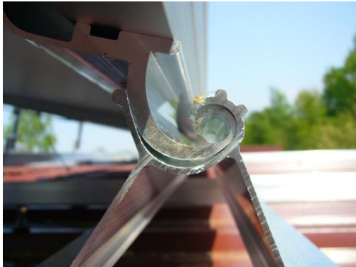
Figure 22 Platform (left) and mounting spiral (right)
