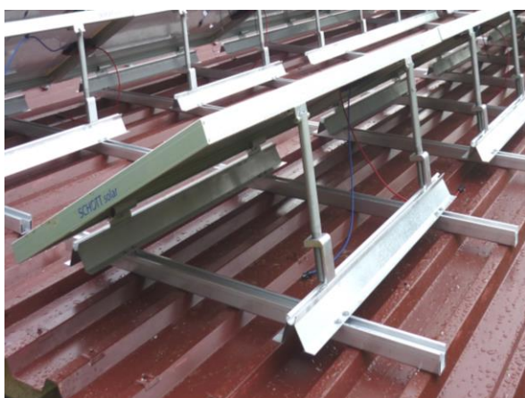
Figure 27 Height - adjustable module support
