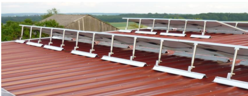
Figure 12 Height-adjustable module supports
