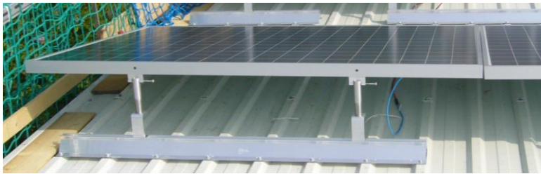
Figure 5 Base profile extension at the verge
