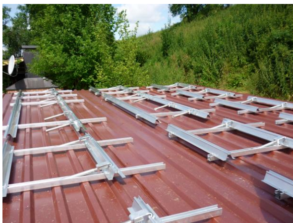
Figure 26 Inserted module support set
