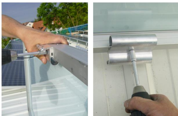
Figure 25 Mounting the module fastener set at the rear (left)
